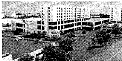
Metro Center Atrium. (Simone Development)
